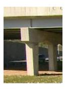
A bridge abutment is a wall supporting the ends of a bridge generally retaining or supporting the embankment under bridge ends and composed of stone, concrete, brick, or wood (includes wing walls).
